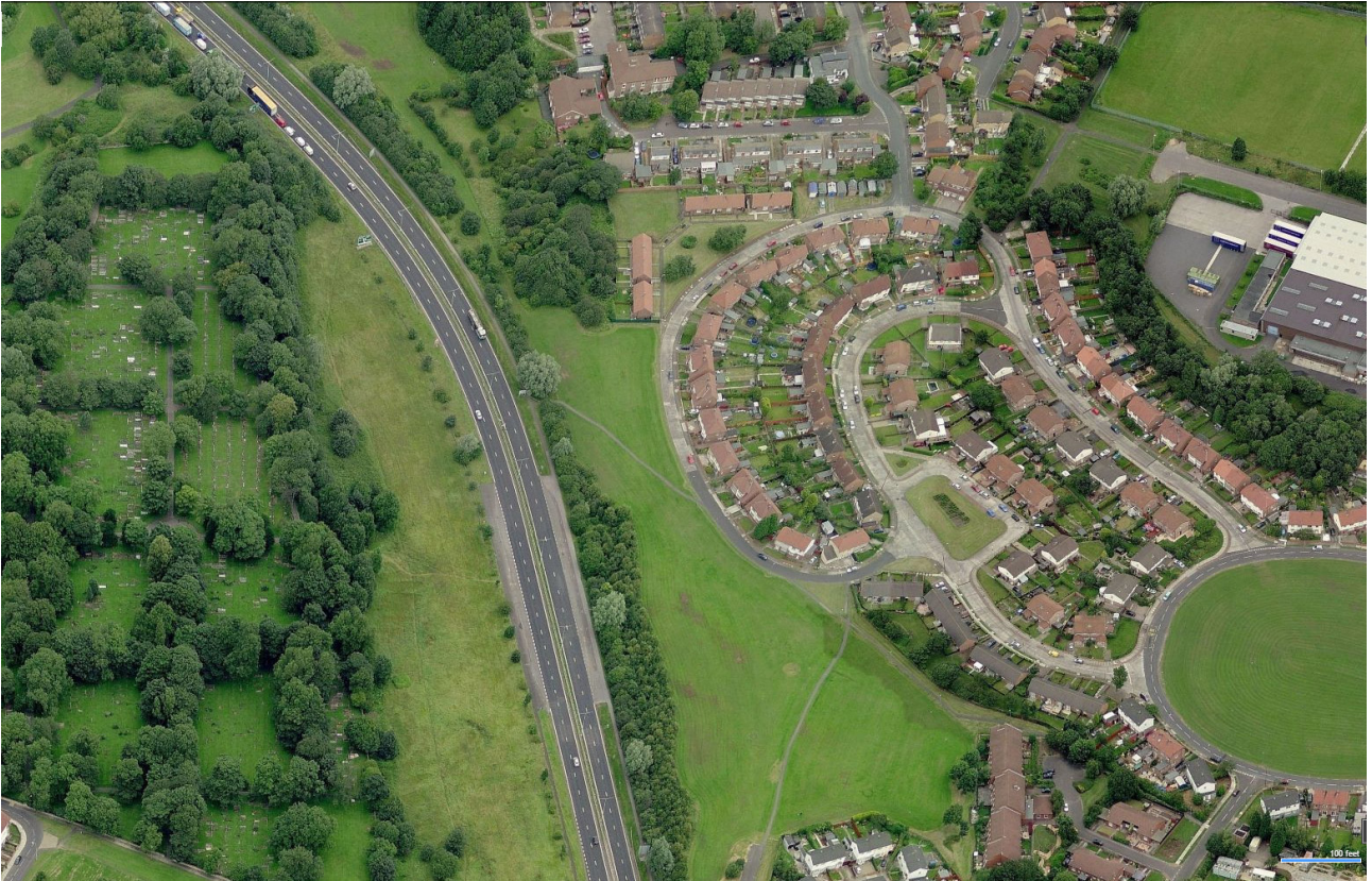
Aerial view of the site showing Falmouth Drive POS to the right, Jarro Cemetary to the left and the larger body of the Salmcombe Ave POS to the lower middle of the image.
